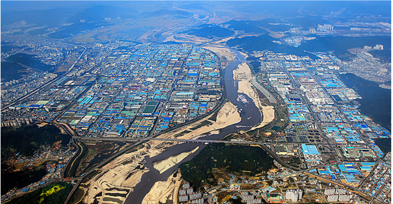
Figure 14: Aerial Photograph of the Gumi National Industrial Complex
